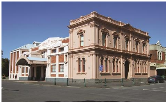
the exterior of Theatre Royal, Camperdown
